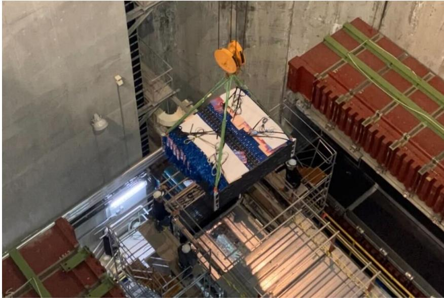
**Figure 3.9.** SuperFGD being installed in ND280 with a crane.
